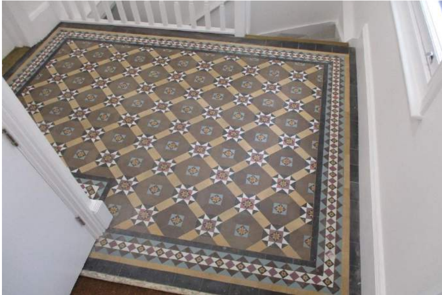
13. Existing mosaic refurbished in entrance lobby
