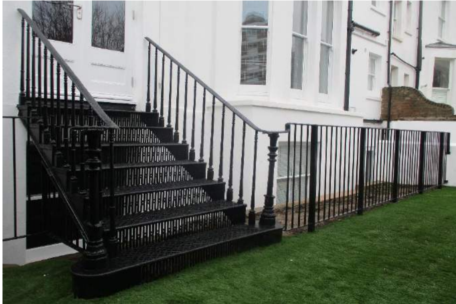
9. Sandblasted rear original staircase
