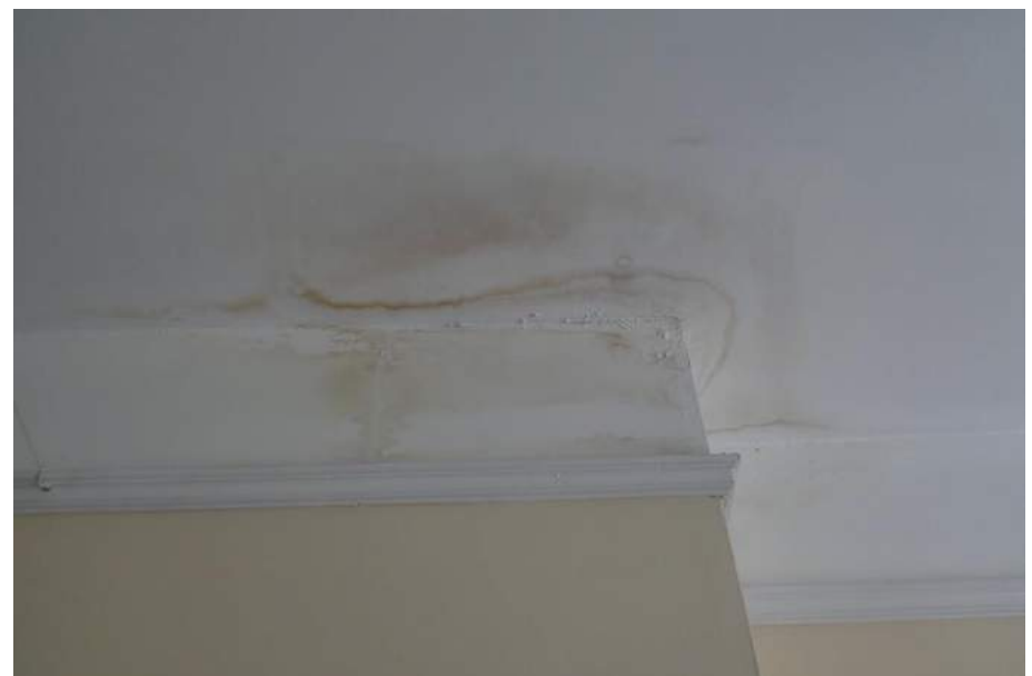
8. Water ingress from roof
