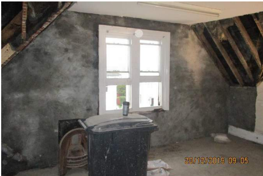
3. New cementitious waterproof membrane
