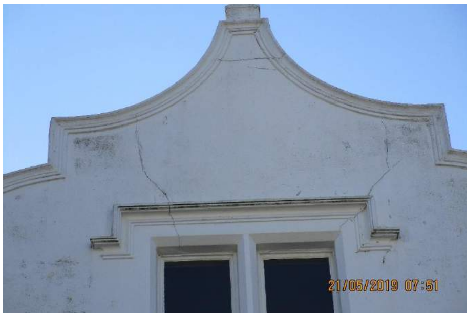
1. Deteriorated render and decorations
