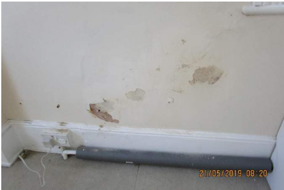
7. Water penetration defects
