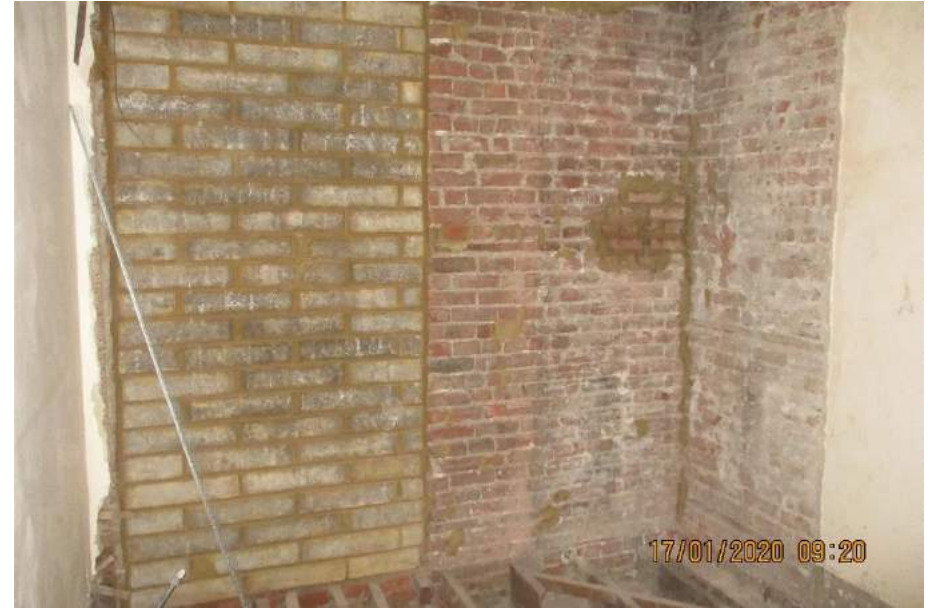
2. Removal of decayed plaster
