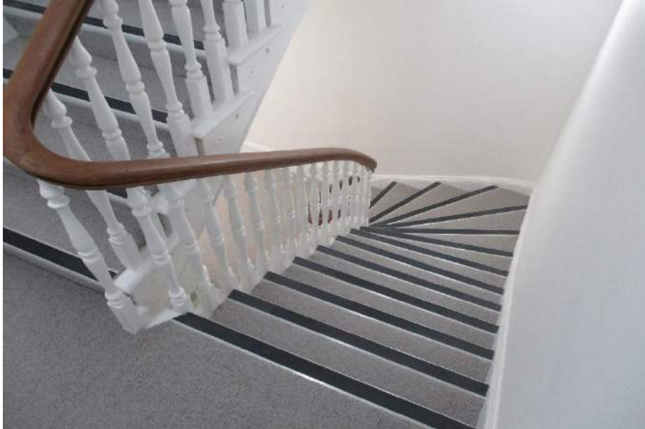
17. Original staircase refurbished
