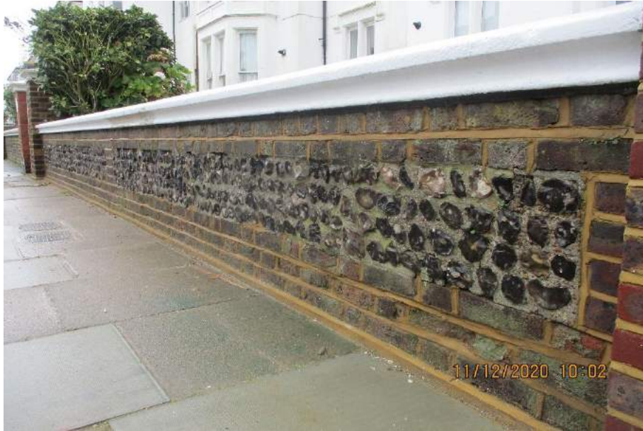
5. Repaired flint wall to front boundary
