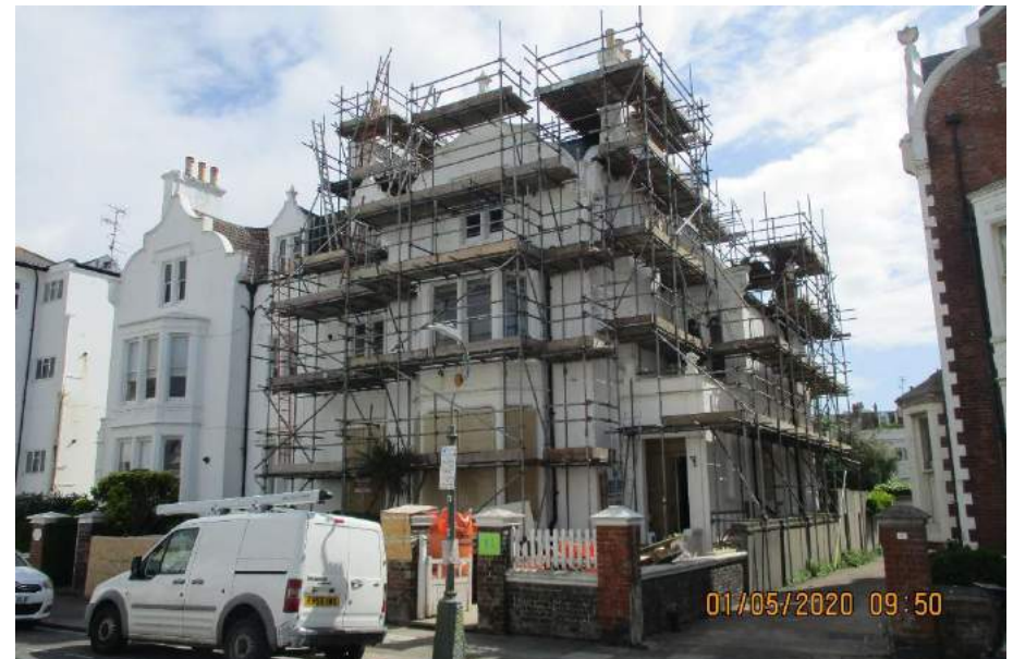
11. Repairs and redecoration to front and flank elevations
