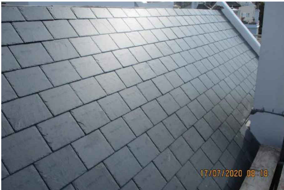
3. Renewed slate roof coverings
