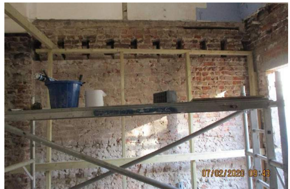
8. Treatment and replacement of dry rot affected timbers
