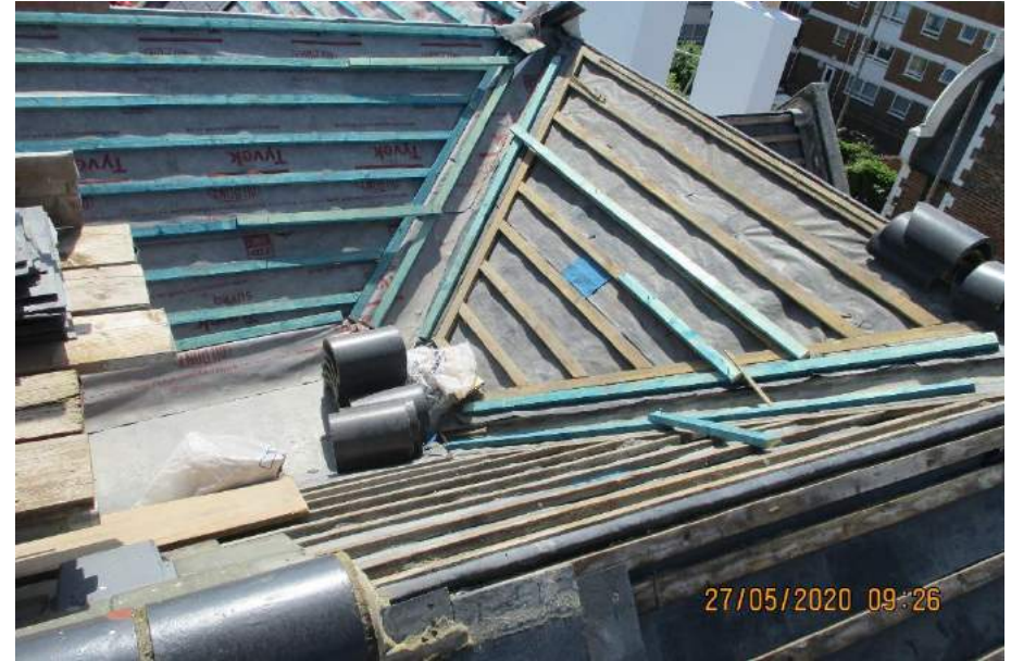
10. Renewal of roof coverings
