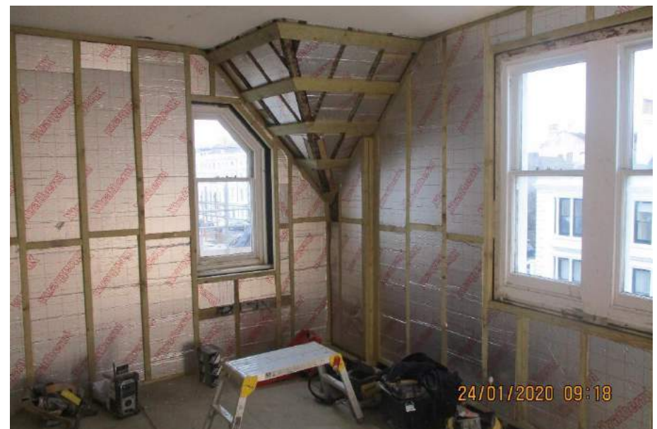
4. Thermal upgrade of external walls
