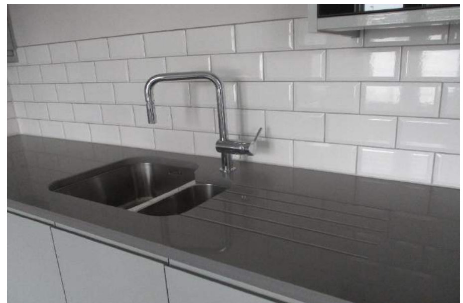
31. Recessed sinks with bevelled drainboard worktops
