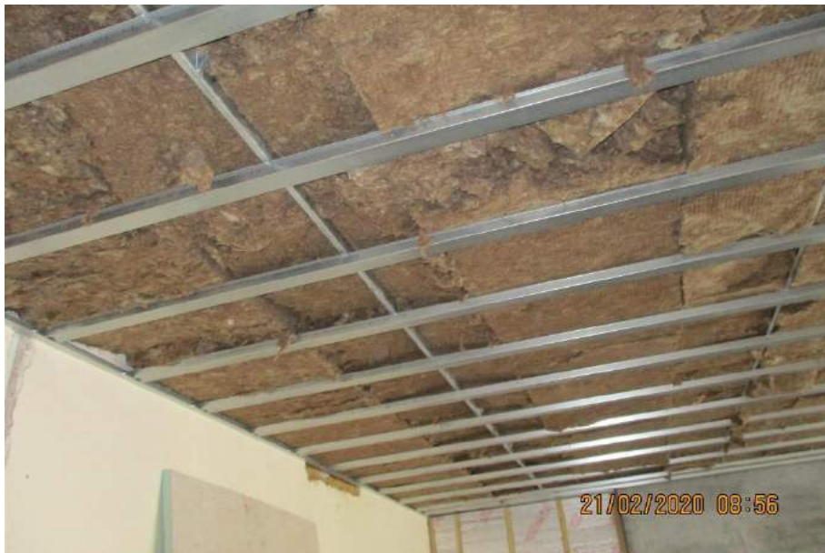
7. Thermal upgrade to ceilings
