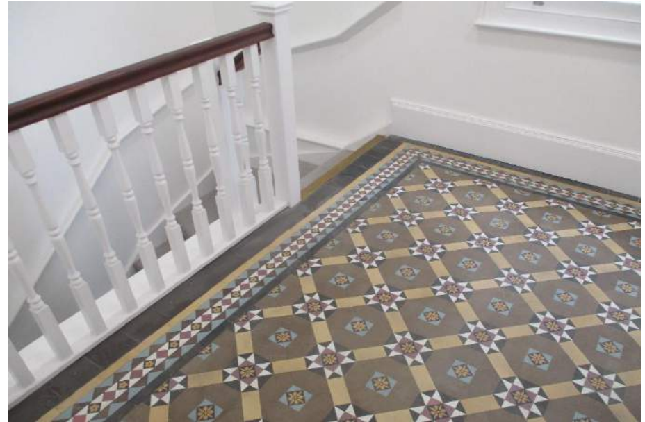
14. Mosaic taken up and re-formed around new staircase
