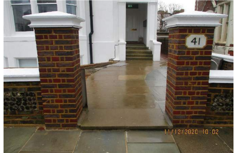
6. Re-constructed entrance piers
