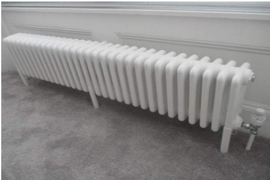
23. New under window column radiators to enhance period feel
