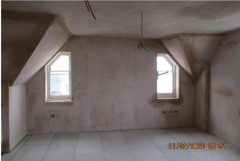
5. Plastering of walls
