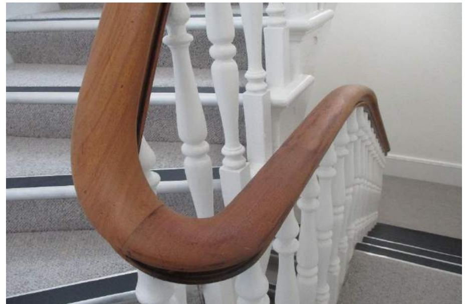
16. Original handrail refurbished
