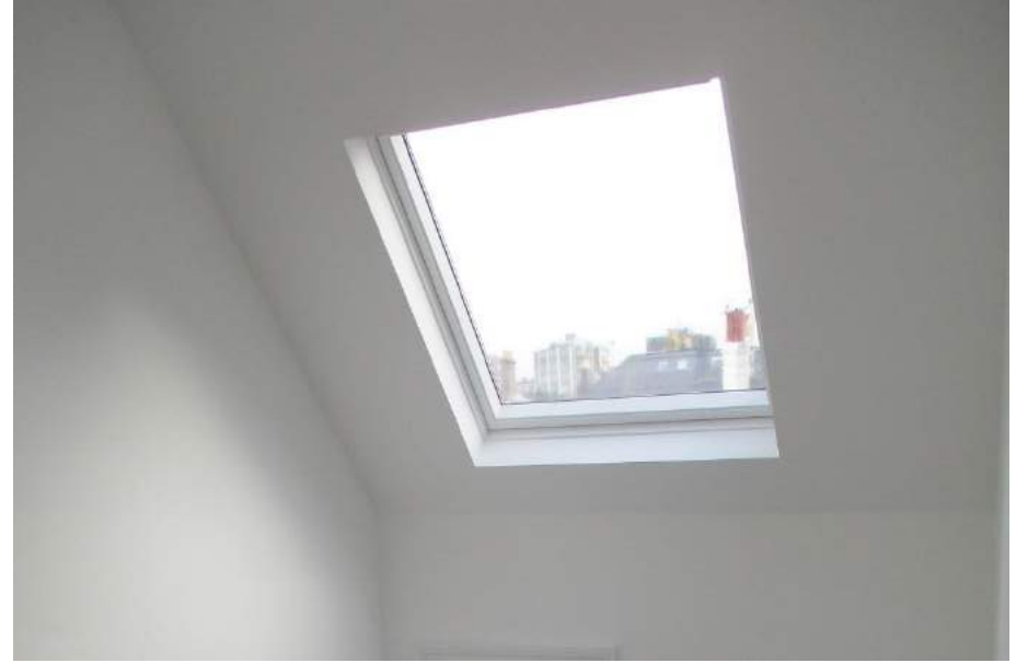
18. New AOV to comply with fire regulations
