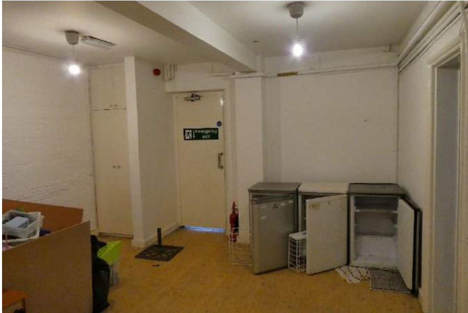
5. Poor natural light in basement
