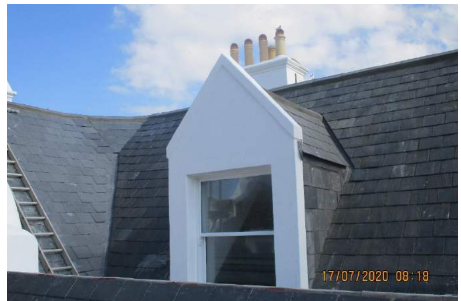
4. Renewed slate roof coverings
