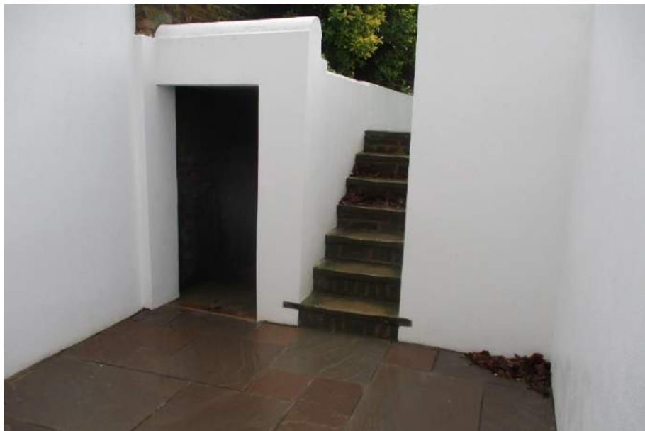
11. Basement flat courtyard
