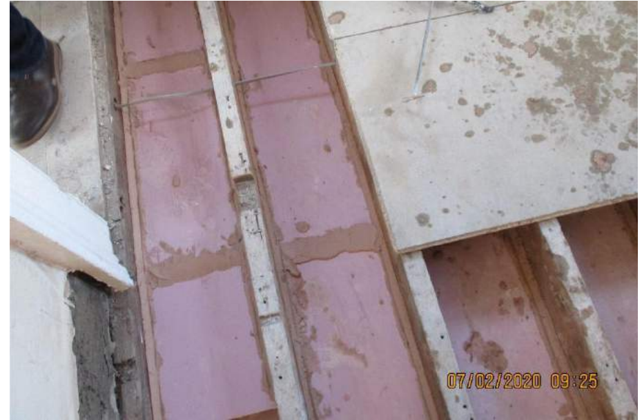
6. Fire compartmentation to separate floors
